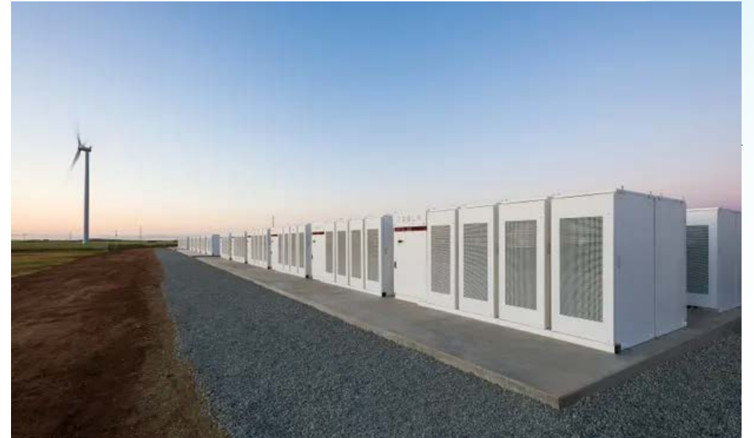
The Hornsdale Power Reserve. A capacity of 129 MWh installed in Australia by Tesla.
